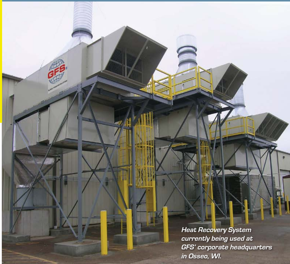
State-of-the-Art, Air-to-Air Exchanger Design, Combined with High Efficiency Direct Fired Air Make-Up Heater.
